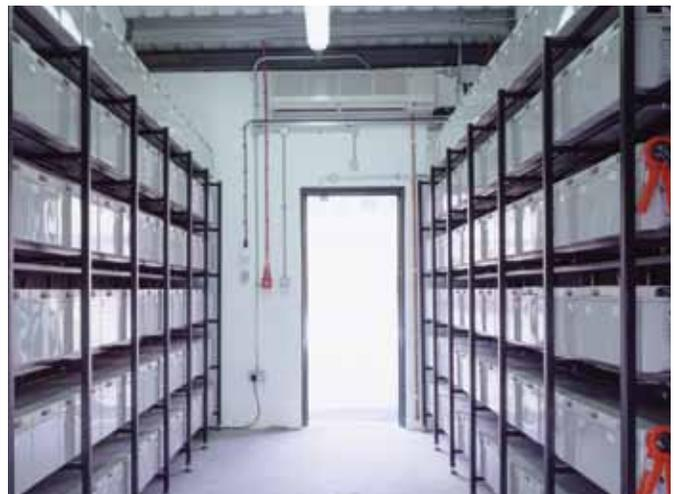
**Eaton Cellwatch battery monitoring system monitors key performance indicators for each individual battery to provide adequate time to detect and replace a bad battery, mitigating the risk of downtime.**
